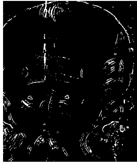
Figure 6. Crack Map after supervised classification
