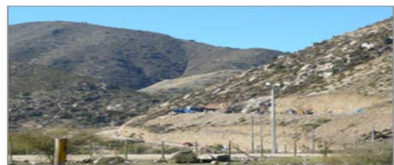
Erosion near a mining road, Pelambres mine, Chile PHOTO: Rocio Avila Fernandez
